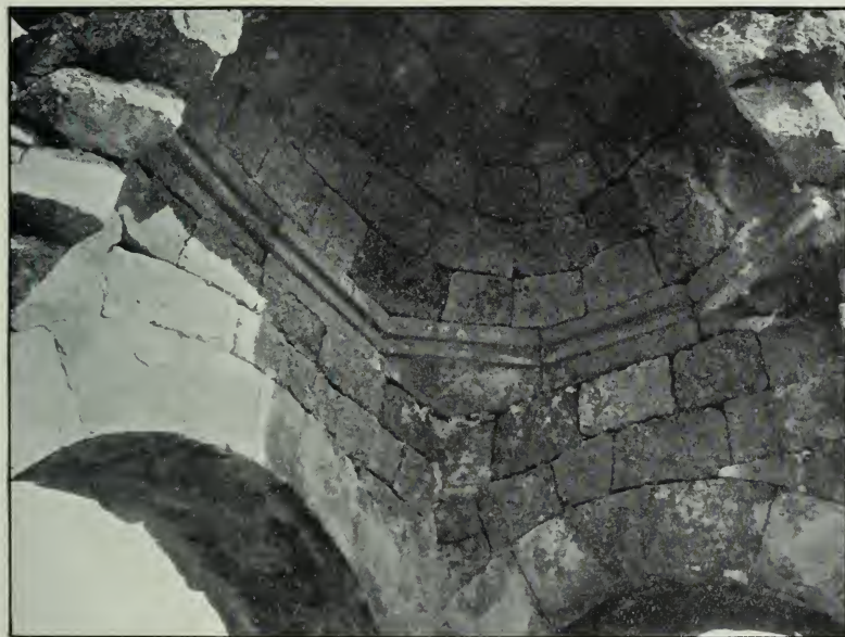
FIG. 42.—Dome of No. 9.
